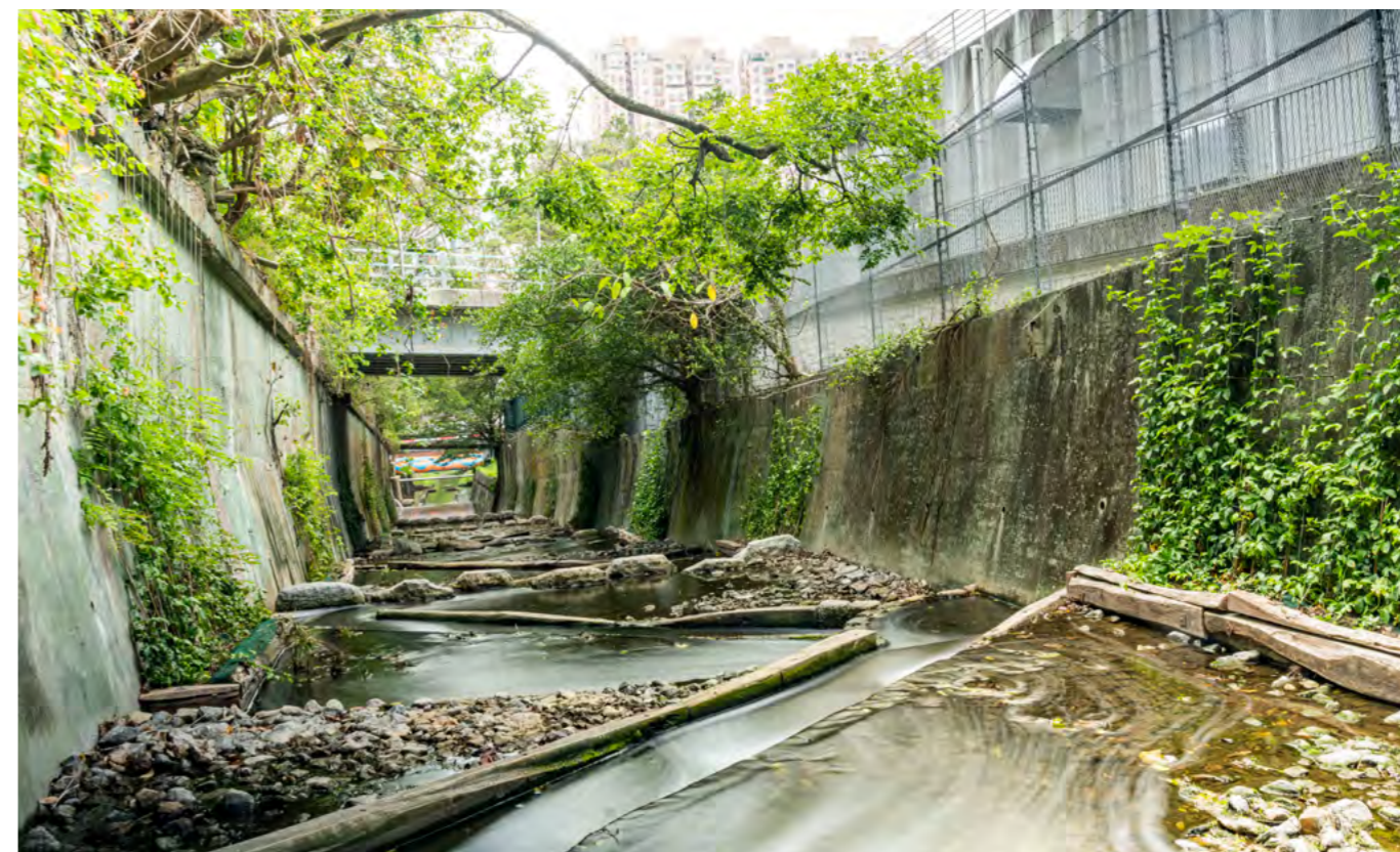
Jordan Valley Channel Revitalisation
